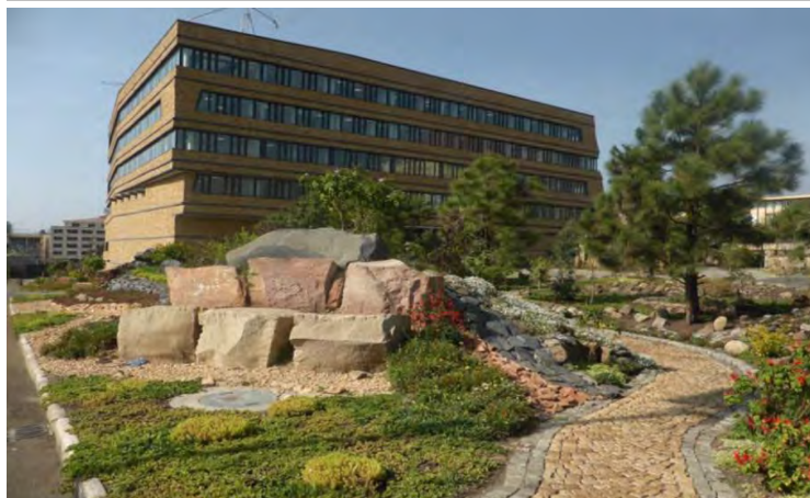
The new Julius Nyerere Peace and Security Building of the African Union Commission holds the plenary hall for the AU Peace and Security Council as well as the AU’s situation room and operations room; the building offers working space for more than 300 employees.
